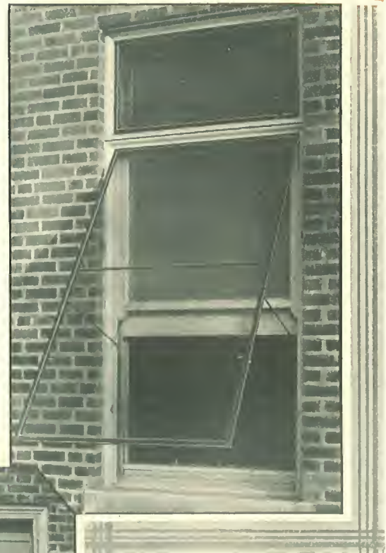
(Above)—Screen is held open with stay rods for window washing. At the top are pivot hinges, one fixed, the other operated by a small inconspicuous trigger which is easily released when the screen is taken out for storage. Spring latches lock the screen at sides.
